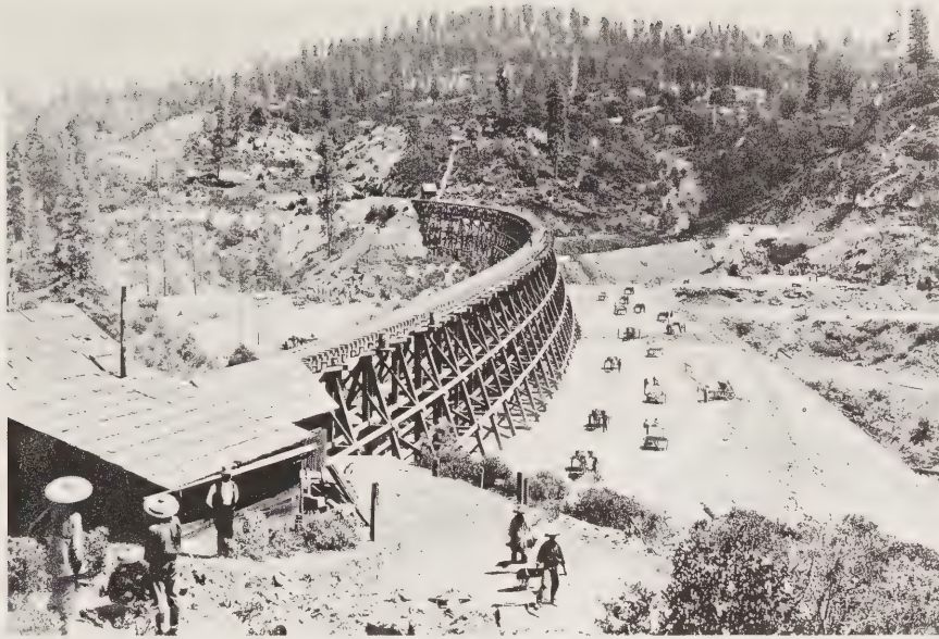
Chinese Laborers Filling Dirt Around a Wooden Trestle in the Sierra Nevada Mountains, Using One-Horse Dump Carts and Wheelbarrows
